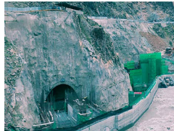
Dasu Hydropower Project
