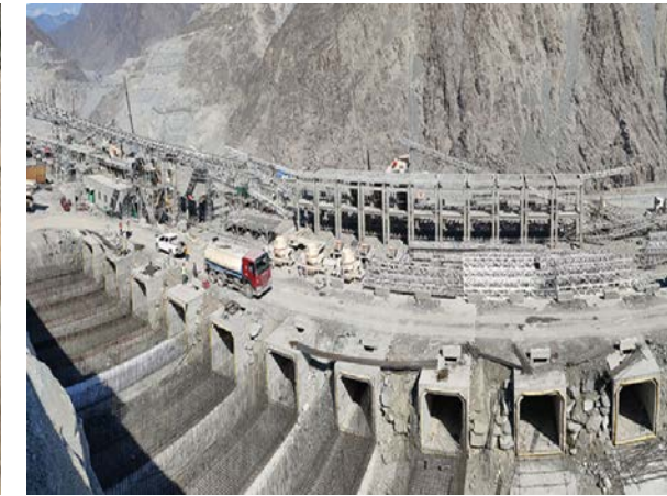
Diamer Basha Dam
